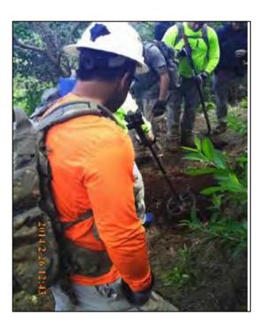
Photograph F-56: Confirming excavation is clear of anomalies prior to backfill. Remedial Investigation Report, Pali Training Camp, Oahu, Hawaii
